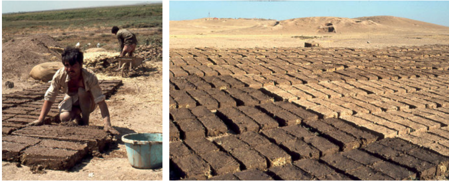
Fig. 6: The images here show the production of bricks in molds by Syrian laborers preparing to build a 1982 addition to the excavation house of the German mission to Tell Bi'a near Raqqa (courtesy K. Englund).
