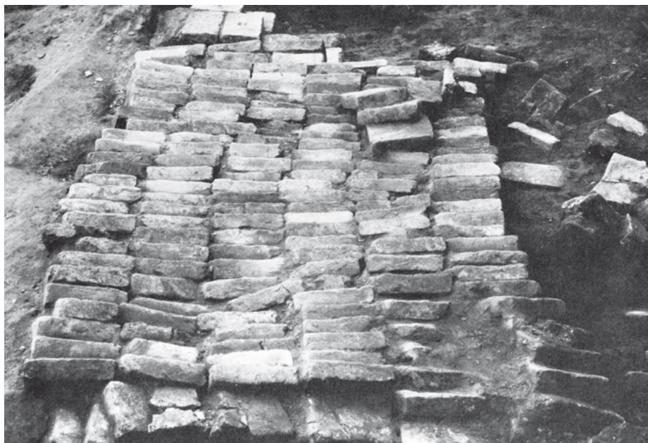
Fig. 9: Piles of bricks left over from the building of Shulgi's mausoleum (taken from Woolley 1974, pl. 2b).
