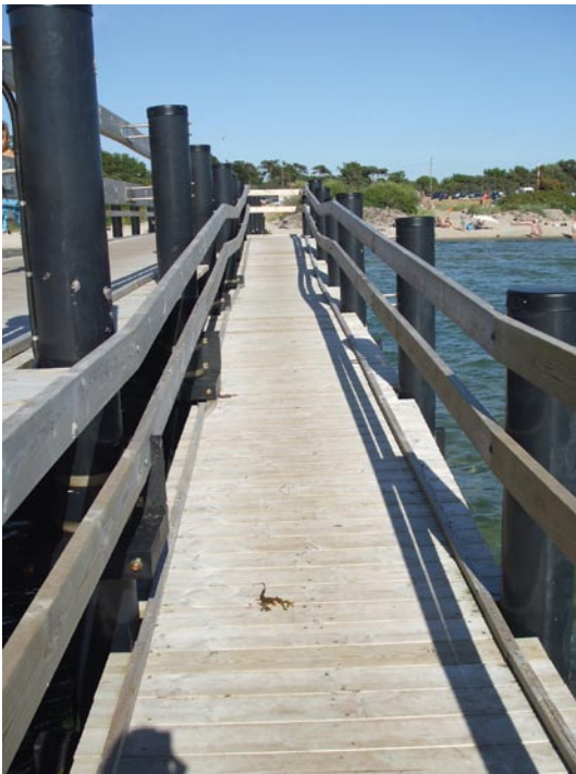
Figure 9. & 10. The jetty is a wood construction with safety railings and edges, and the underwater part is a metal construction
