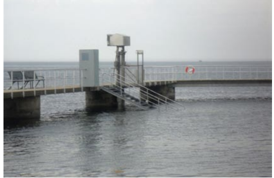
Figure 7. & 8. Access to the water via from a wooden jetty via ramp, staircase and pool lift
