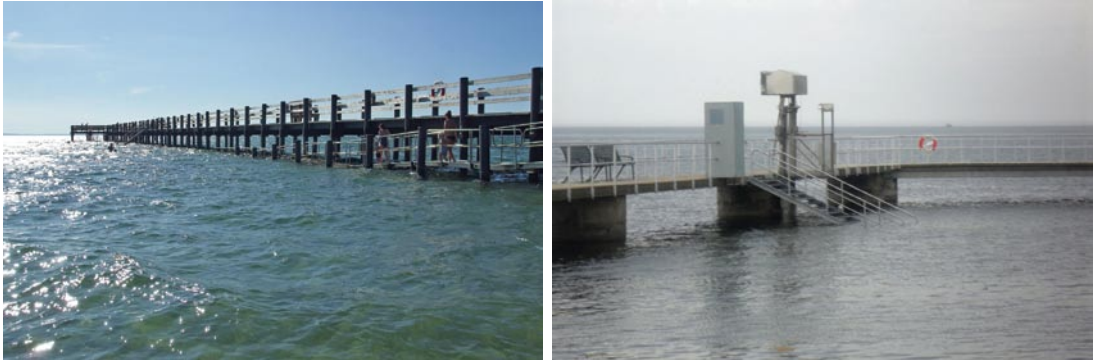
Figure 7. & 8. Access to the water via from a wooden jetty via ramp, staircase and pool lift
