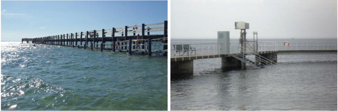
Figure 7. & 8. Access to the water via from a wooden jetty via ramp, staircase and pool lift
