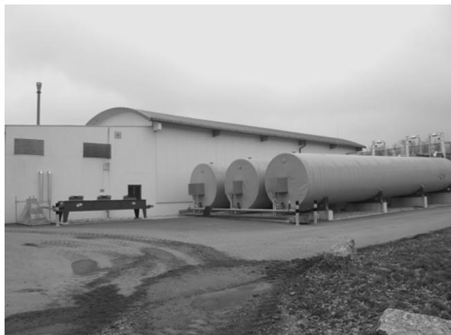
**Photo 2.** A view of steel tube fermenters<sup>8</sup> (right part of photo) – BGS Amstetten (Austria) – photo by authors
