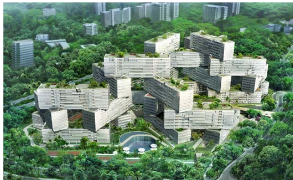
Fig 3. Example of complex apartment building
