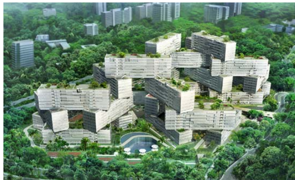
Fig 3. Example of complex apartment building
