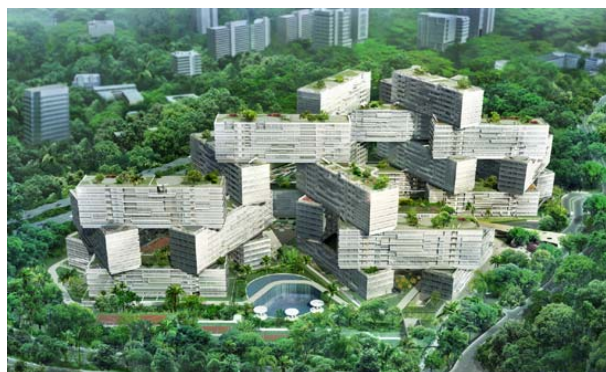
Fig 3. Example of complex apartment building
