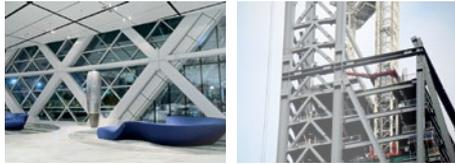
Intumescent fire protection is used on the architecturally exposed steel structure of Capital Gate. The exposure of the members and their connections is a very important aspect of the design and so an intumescent coating was the applicable choice.
