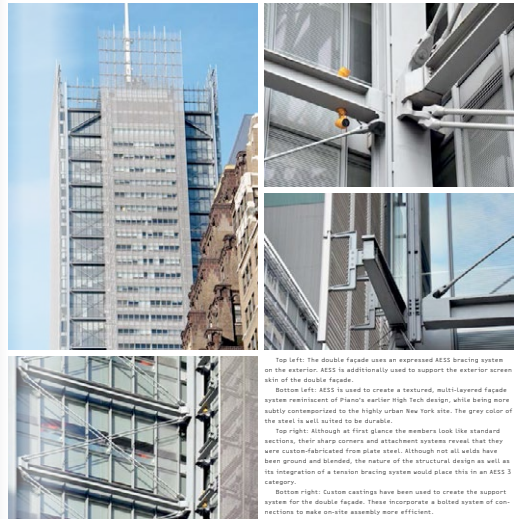
Bottom right: Custom coatings have been used to create the support system for the double facade. These incorporate a bolted system of connections to make on-site assembly more efficient.
