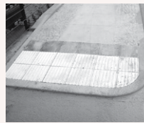
Abb. 3.3.10 Sidewalk with wheelchair-accessible curb ramp (1:10 slope, minimum surface, and direction field as a hand-casting point for wheelchair users as well as blind and visually impaired persons
