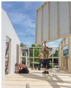
Fig. 516 External walls, 12 cm light earth, internal walls with stacked earth bricks
