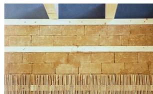
Fig. 240 Dry laid bricks with reed plaster lath (Paproth)
