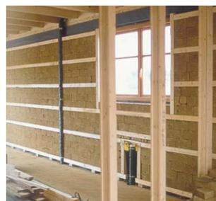
Fig. 239 Prefabricated timber frame house with stacked earth brick internal wall lining (Paproth)
