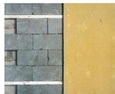
Fig. 242 Stacked internal wall lining (see project 2)
