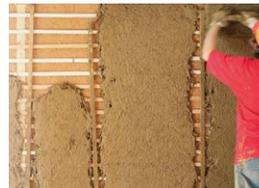
Fig. 204 Manual application smoothed with a float. The thickness of the vertical lath determines the thickness of the plaster. Closing the gaps with the same material
