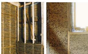
Fig. 202 Woodchip light earth internal wall lining compacted behind reed plaster lath as lost formwork
