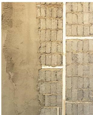
Fig. 238 Stacked internal wall lining in timber frame panels coated with a layer of undercoat plaster (see project 9)
