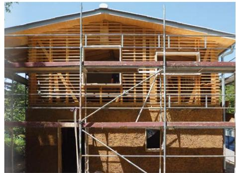
Fig. 517 Continuous application of light earth on battens under the already complete roof with larch wood window jambs already in place
